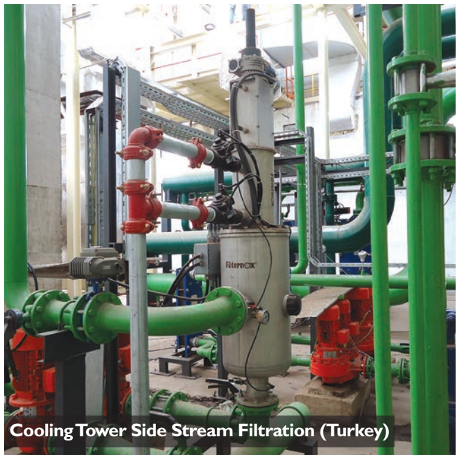
Glass Industry, Cooling Water Filtration (Turkey)
